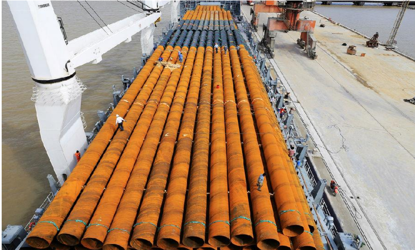
SUPER LENGTH PIPE PILING LOADED INTO M.V.
