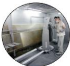
6. Painting antirust paint
