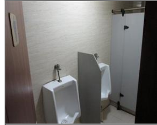
Photo of the sanitary facilities Toilet.JPG
