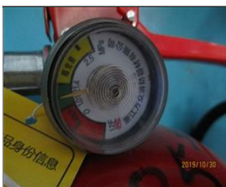
Photo of fire safety equipment Fire extinguisher pressure was OK.JPG
