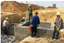
Liquid level inspection of collection well and biochemical pool
