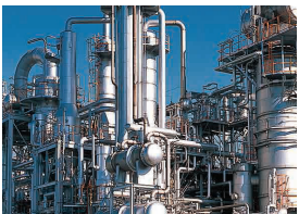
Industry Liquid level inspection of chemical container
