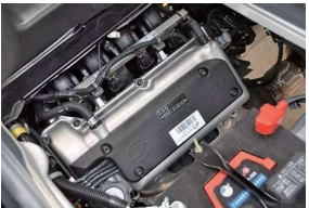
Temperature detection of machinery and equipment
